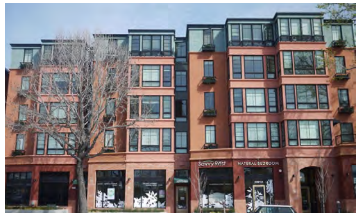
The developer of this 38-unit property in Berkeley, California, provided seven affordable units in exchange for an extra story.
