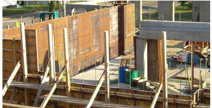
Ripley Gardens construction, Minneapolis
